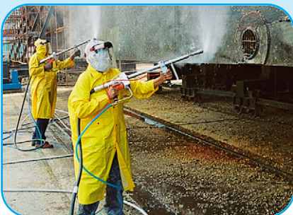
Twin gun surface preparation
