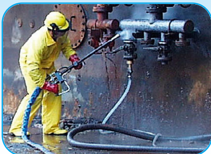
Surface preparation of valve manifold
