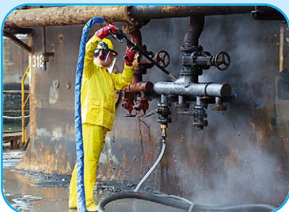
Surface preparation of intricate pipework
